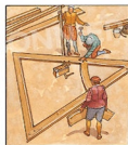
The long and expensive oak timbers needed for the framework were cut and fitted at the builder's yard.
