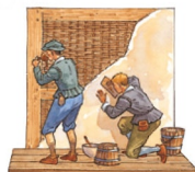
Completing the theatre walls
