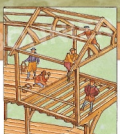
Carpenters on site re-erected the frame by matching the marks. The timbers were joined with wooden dowels.
