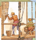
The frame of the theatre was filled with wattle and plastered over. The building appeared circular but was actually formed of many short sides.
