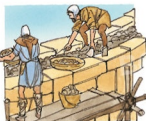
The walls were made like a sandwich – fine-trimmed blocks were used on the inside and outside surfaces and the middle was filled with a rough limestone rubble concrete.
